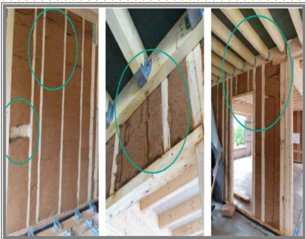
POSE NON JOINTIVE DE PANNEAUX
